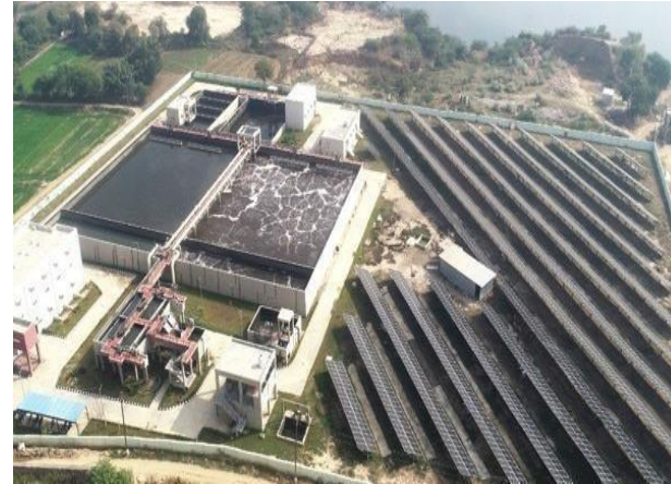
30 MLD STP Kota Rajasthan(Includes Solar Plant)
