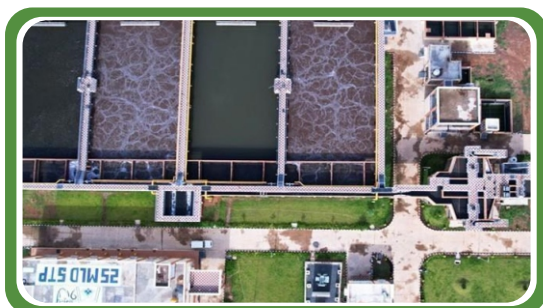
25 MLD STP, Jagdalpur, Chattisgarh
