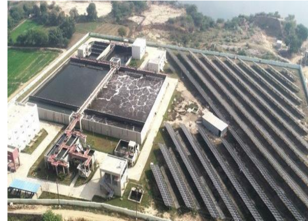
30 MLD STP Kota Rajasthan(Includes Solar Plant)
