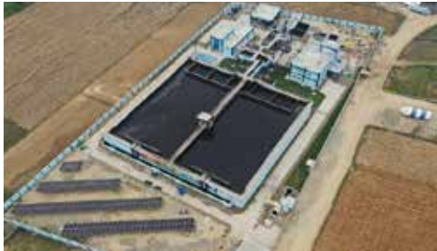
42+20+1 MLD Bareilly UP (includes solar plant)
